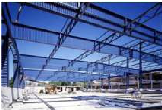
Fig. 2: Single storey building. Corrugated web beams
