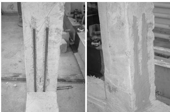
Steel bars in slits      Resin applied in the slits
