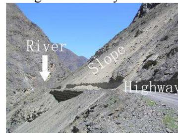
Fig.1 Debris flow at the 616<sup>th</sup> km along Mt. Tianshan highway, Xinjiang, China
