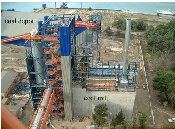
Fig.1 Coal mill and a coal depot in the cement factory
