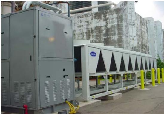
Figure 6. ORC power plant using gas turbine exhaust in East Hartford CT
