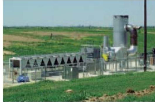
Figure 7. ORC power plant using landfill flare exhaust in Austin, TX
