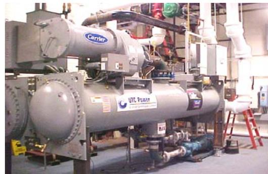
Figure 9. Water-cooled, hot-liquid driven ORC power plant in East Hartford, CT
