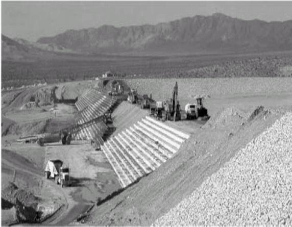
Fig.1 Schematic of stepped spillways
