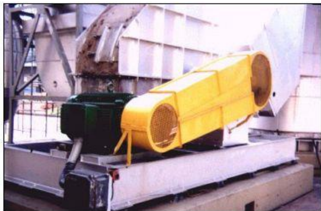
Fig. 13. Resized 75 hp high-efficiency motor.
