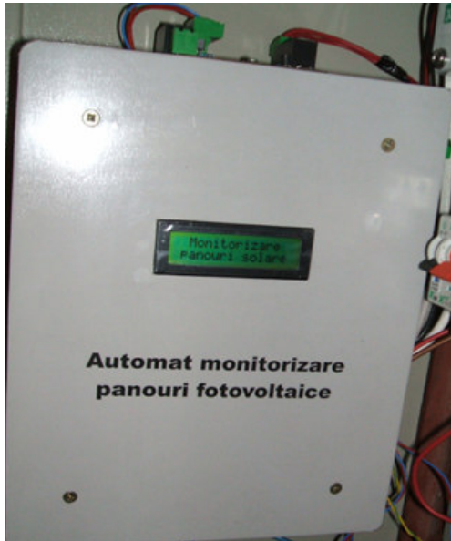
Fig. 20 Automat for panel orientation and for monitoring the movement of energy
