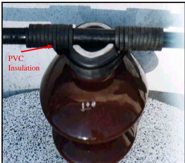
Fig.10. Application of PIC insulation as tie wire
