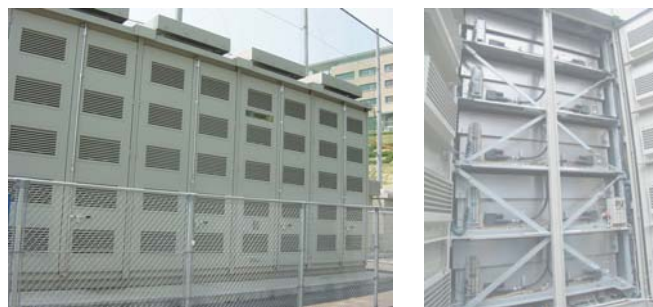
Fig.1 Appearance of NAS battery in Campus
