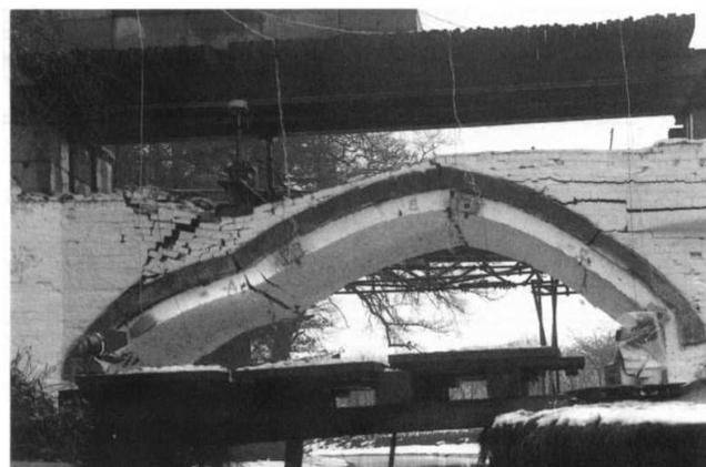
Figure 4: Collapse of the Bridgemill arch bridge. (Source:[http://archive.niees.ac.uk/talks/dem/nenad\\_bicanic.ppt](http://archive.niees.ac.uk/talks/dem/nenad_bicanic.ppt))
