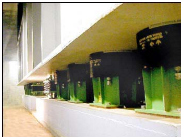
Fig. 3 Mounting viscous-elastic system under technological equipment foundation
