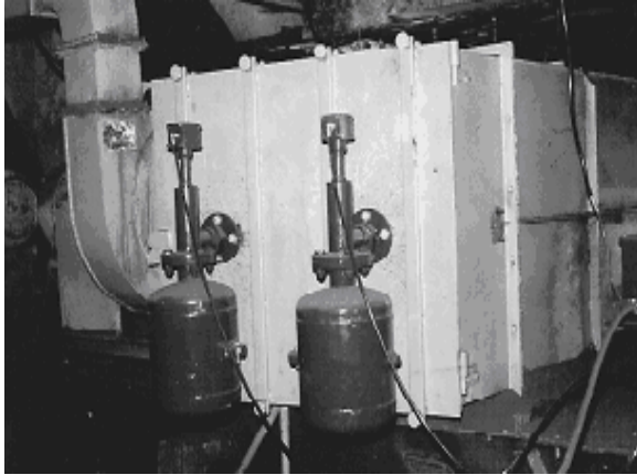
Fig. 4. Small capacity ABD mounted on the wall of coal dust filtration system for belt conveyor in large electro-thermal plants
