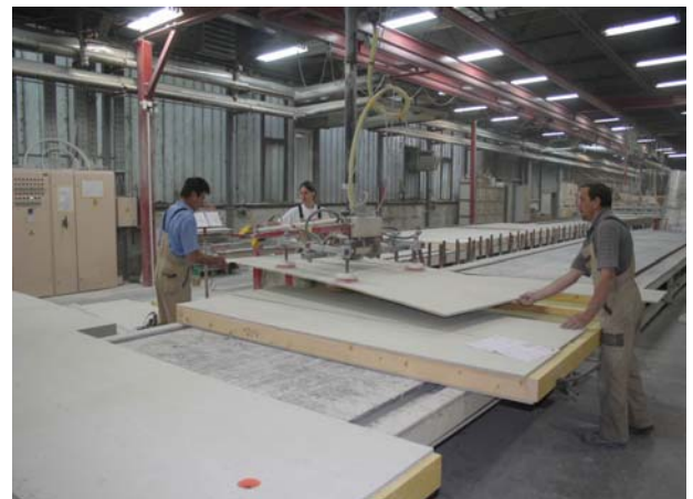
Fig. 1. Factory preparing of prefabricated walls.
