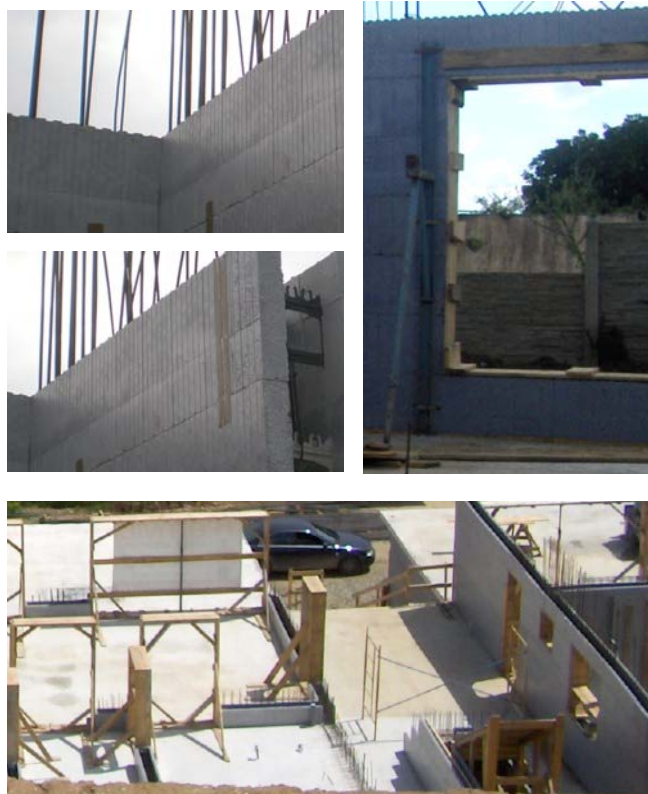
Figure 7. Pictures taken during the installation process (Photo: A.T. Mircea)
