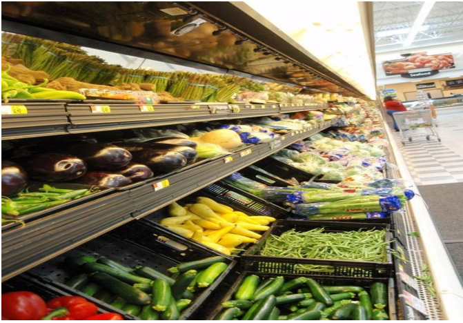
Fig.1 Boxes obstructing the return grille of a refrigerated display cabinet.
