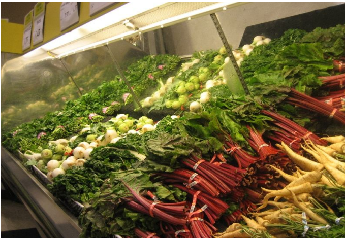
Fig.2 Produce obstructing the return grille of a refrigerated display cabinet.
