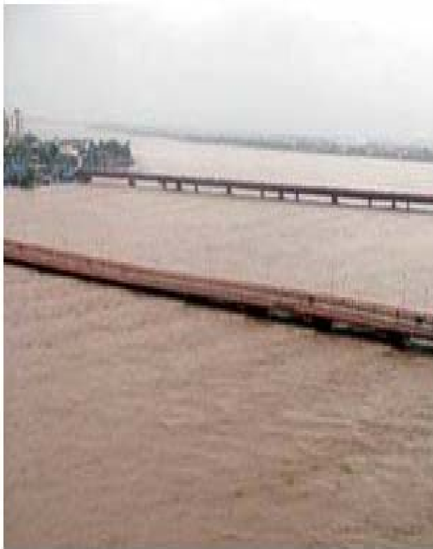
Fig. 7 Overflowing Bridges during Flood
