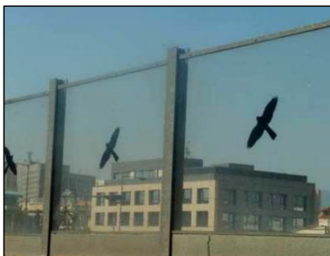
Fig. 20 PMMA transparent barriers in Attiki Odos (2011)
