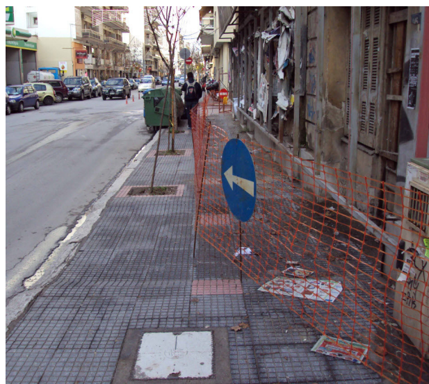
Fig. 5: Low walkable road segment
