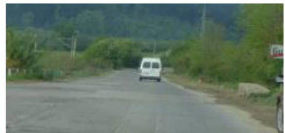
Fig.9 General view of the existing road sector selected for demonstration project[6]
