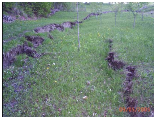
Fig. 9. Landslide from Bezdead (2005)
