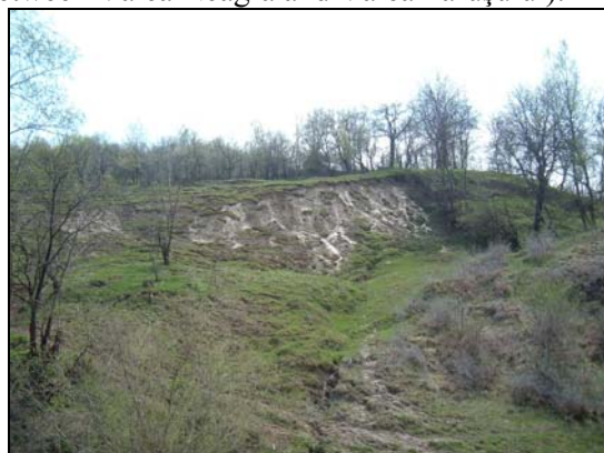
Fig. 10. Landslide in Buciumeni (2005)
