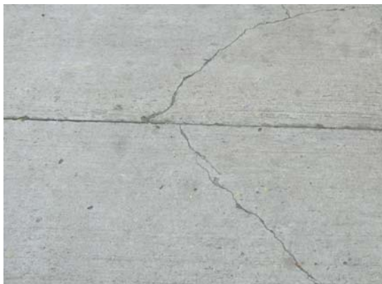
Figure 5. Corner cracks
