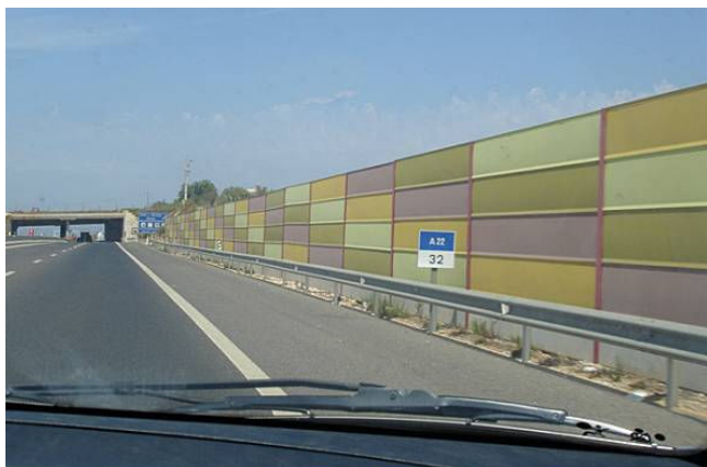
Figure 8- Sound protection systems along the new part of the highway from the A2 connection to Bensafrim (E. Bertè photo)
