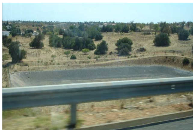
Figure 9- A pond for the collection of polluted water (E. Bertè photo)
