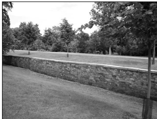
Figure 11 – A portion of the long “Ha-Ha.” It is a military fortification device employed in English landscapes to provide uninterrupted views, while keeping animals, people, and now cars from entering the inner area. (Used by permission of Jon Bryan Burley ©2007, all rights reserved).
