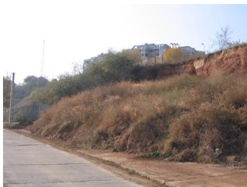
Figure 11. Landslide along the shoreline in Constanta port area
