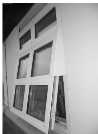
Fig 9: The opening of the window could also be restricted to help the energy conservation in the building.
