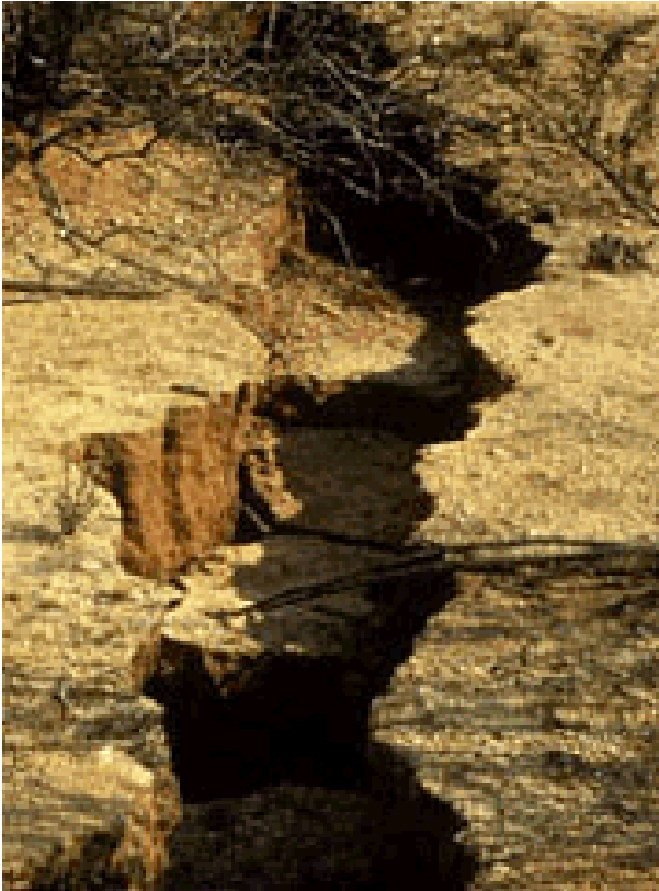
Fig.1. earth fissures caused by differential settlement of Sirjan land
