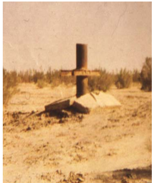
Fig.3.Subsidence around a pumping well in Sirjan
