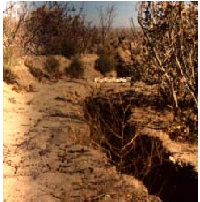
Fig.2. earth fissures caused by differential settlement of Sirjan land
