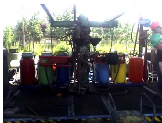
Fig. 5 Removal of all the fluid materials existing on VHL using a SEDA equipment
