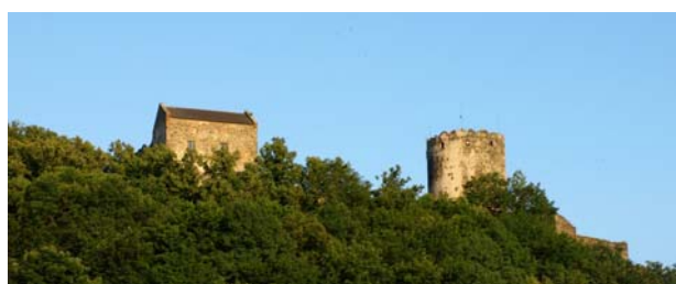
Fig. 8. The Bolków Castle. On the left – residential tower (photo: J. Gubański)
