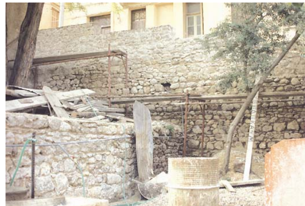
Fig.19 Stone masonry approximately 0.60 m. thick .
