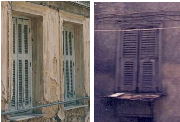
Fig.26 The openings are covered with Venetian blinds.
