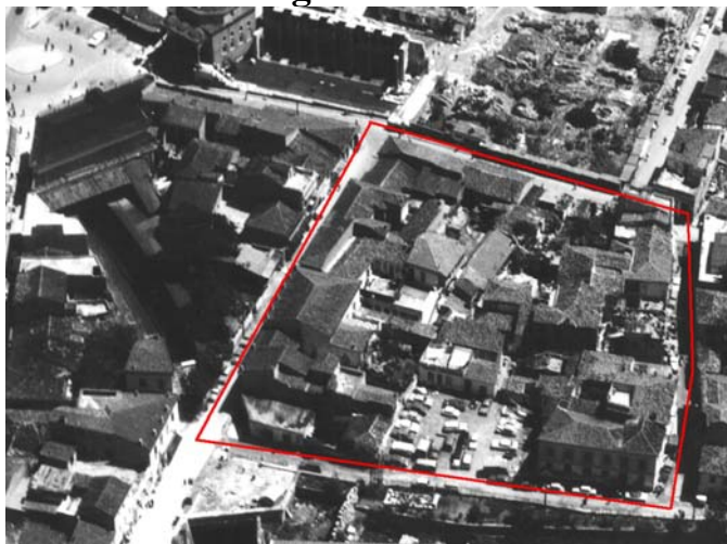
Fig.3 Aerial photo of the historical center of Athens.
