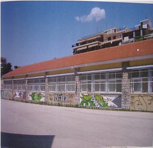
Figure 9. Existing bare grounds
