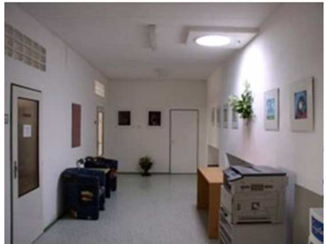
Fig. 7 Photograph of the room with the investigated light guide
