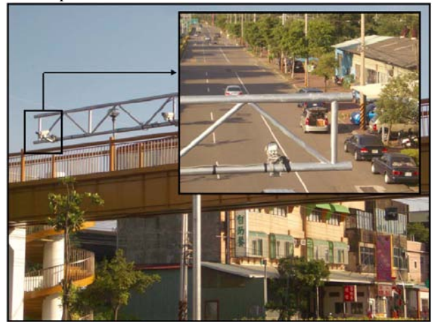
Fig.15 Set up and location of the stationary CCD camera ( H=6 m, \theta=14^\circ , f=8 mm, R_p=6 mm/240 pixels)
