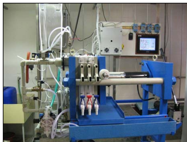
Fig. 13 Filter press workplace – side view
