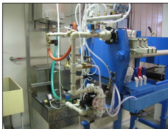
Fig. 14 Filter press workplace – front view
