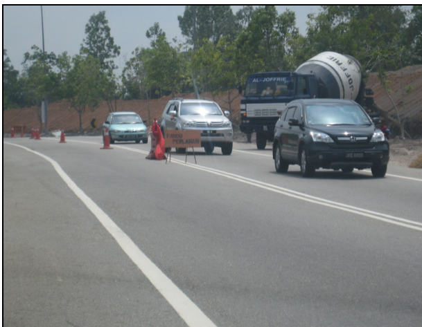
Fig. 3: Two lane road construction site without a flagman to control the safety and smoothness of the traffic flow
