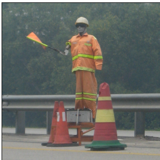
Fig. 9: Automated flagman in a road construction site
