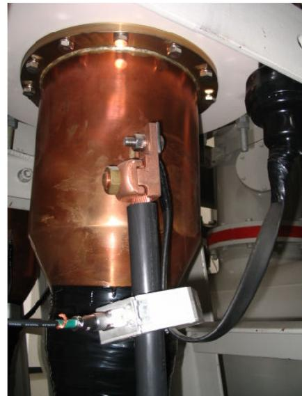
Fig. 2 HFCT installed around the earthing strap of cable termination.
