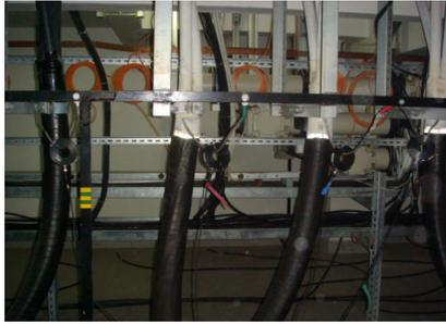
Fig.13 HFCT installed around the earthing strap of cable termination
