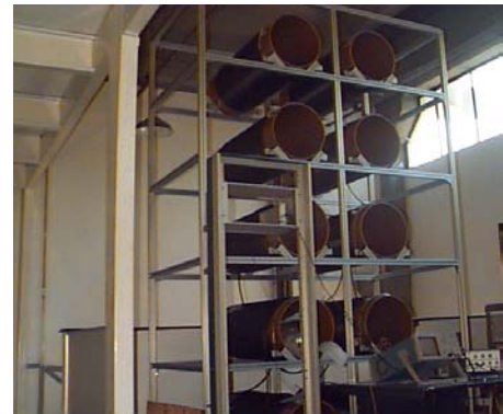
Figure 3. Picture of the pulser structure assembling.
