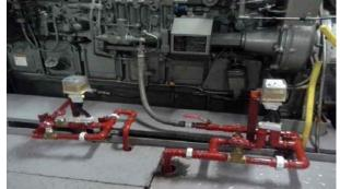
Figure 8. Erection of flow meter (after)
