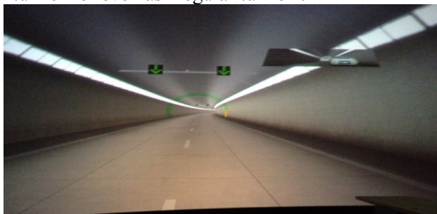
Fig.2: Inside the tunnel
