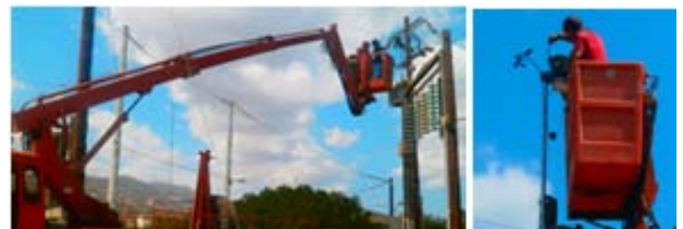
Fig. 5. Installation of the weather station on top of the pollution measurement arch
