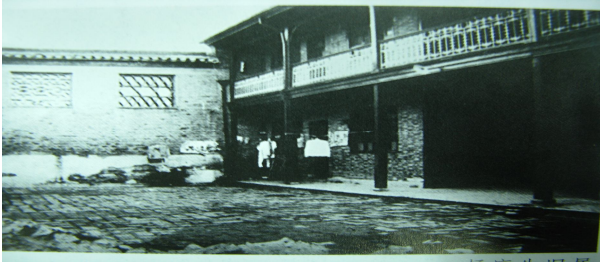
Picture 13: Courtyard of the former residence of Yang Guangsheng
