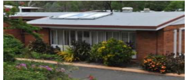
Fig.2: Building 41 at CQUniversity
