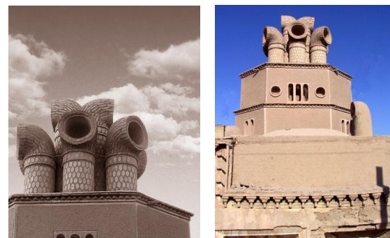
Fig.14: Pipe like wind-catcher(Chopoghi)in Sirjan
