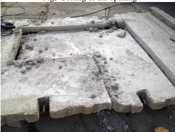
Fig.4 Opening completely cut-out
