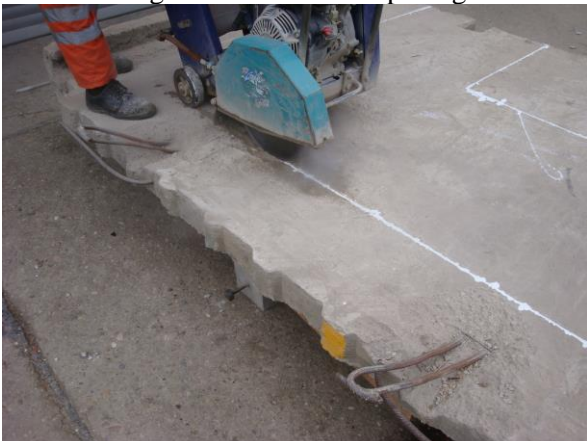
Fig3 Cutting of the opening
