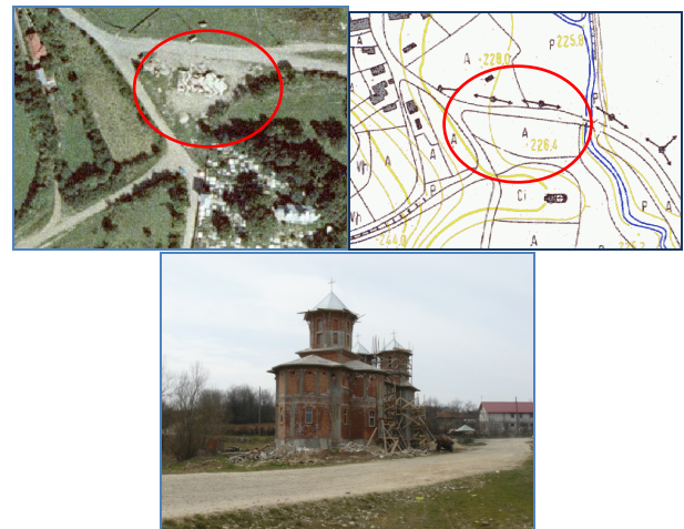
Fig.10 In 2009 the church was in final stage of construction (the moment of checking in situ);
