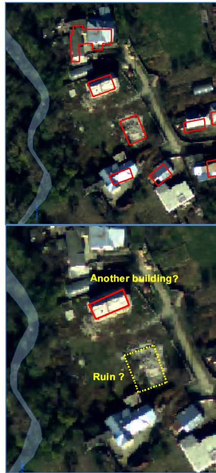
b) Two houses : orthophoto map from 2012 (a new reference background used for check errors);
