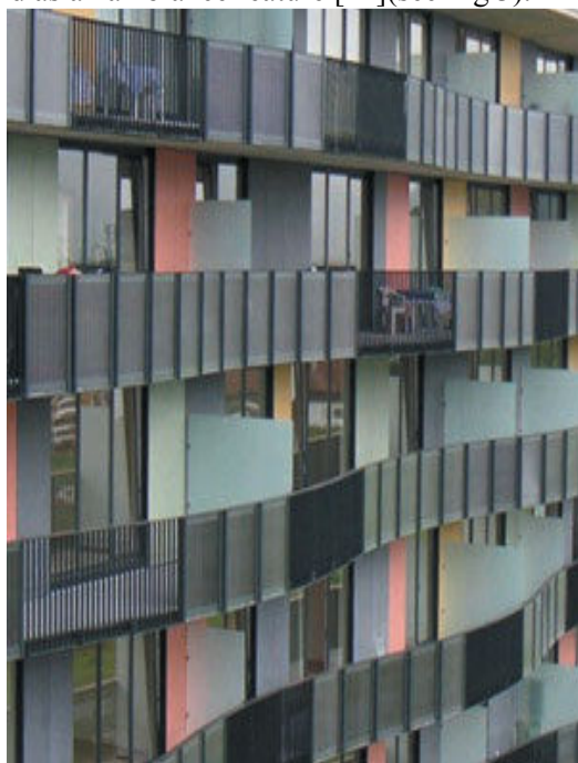
Figure 3 Balconies function as shading device
