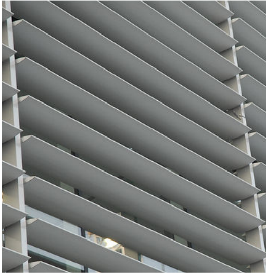
Figure 6 Fixed Louvers are very common in developed countries
