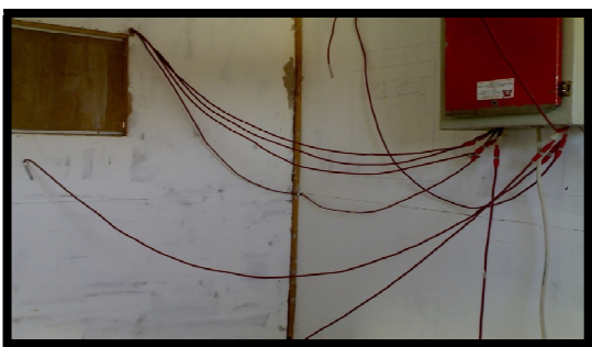
Fig.2 General View of the experimental set-up of the test room and the Trombe wall system
