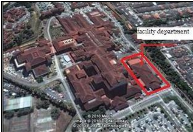
Fig. 1: General view of field study (facility department of HUKM)
