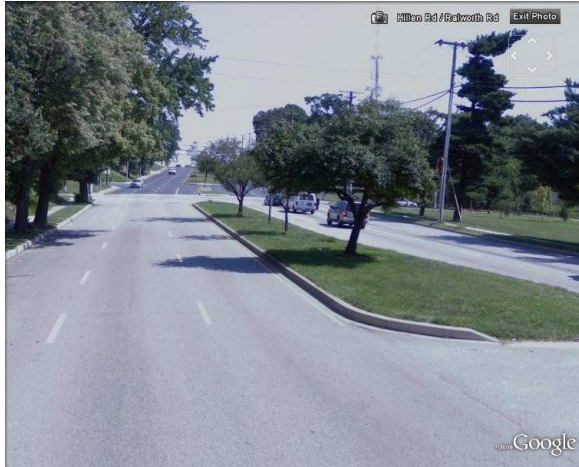
Figure 10. A Sample Road Stretch showing Road Width
