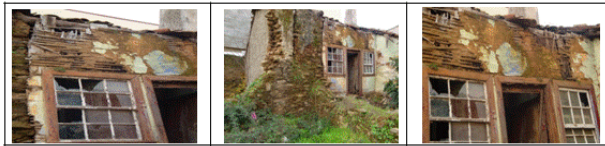
Fig.3 - Appraisal form filled for an example of a tabique construction existing in Macedo de Cavaleiros Municipality (November 2009)
